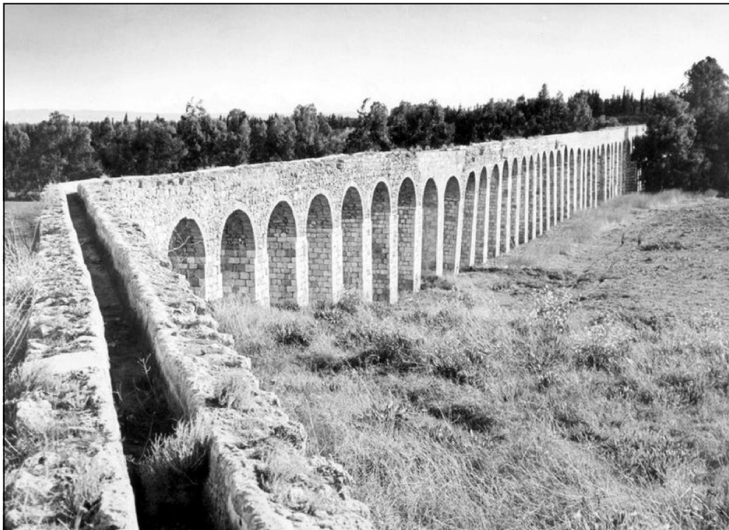
The 'Akká Aqueduct after it was repaired.
